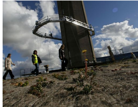
Figure. 2 Rosemarie Andolino, executive director of the O'Hare Modernization Program, center, gives a tour of the 10,000-square-foot vegetated green roof atop the new north air traffic control tower's base building.
