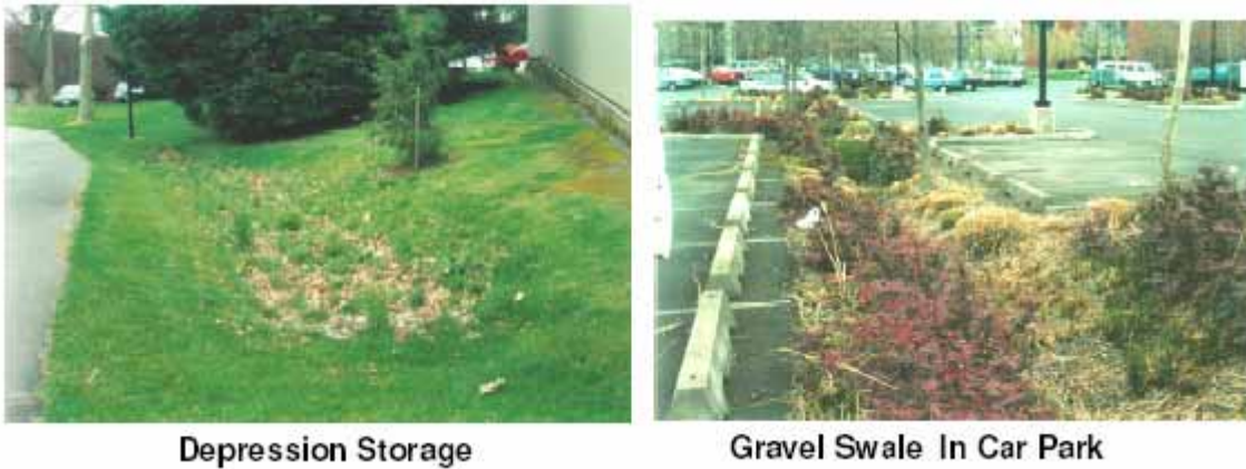
Figure 1. On-site stormwater management measures applied in Auckland, New Zealand
