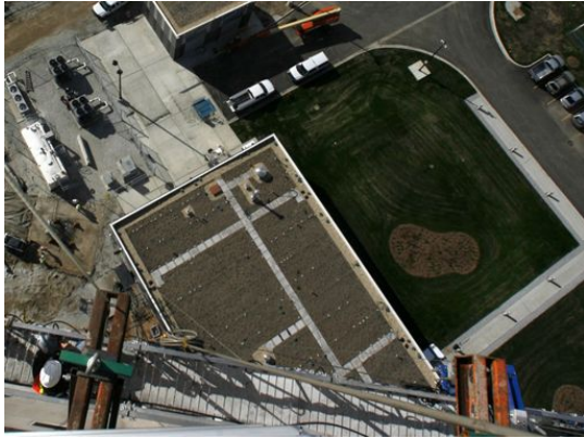
Figure. 1 The new north air traffic control tower's base building at O'Hare International Airport has a 10,000-square-foot green roof.
