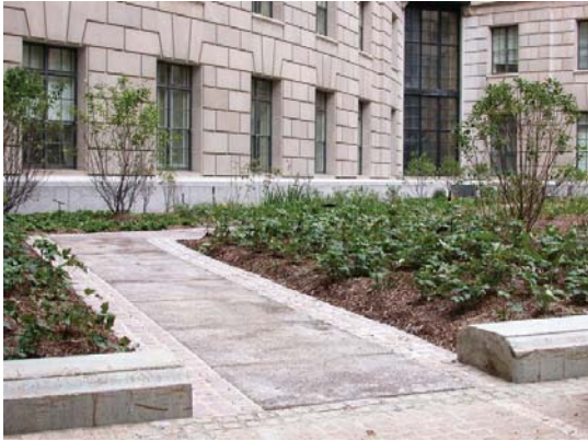
Figure. 1 Porous concrete walkway and rain garden at Ariel Rios South Courtyard.
