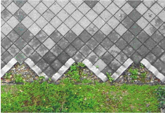
Figure.7 Permeable Pavement in Front of the Design Hall
