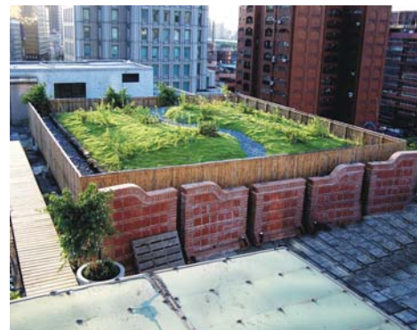
Figure.10 View of Eco-Balcony
