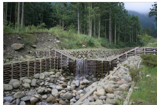
a) sabo dam made of Japanese Fir just finished on Feb 8 2006 b) after the heavy rainfall event on Jun 26 2006
