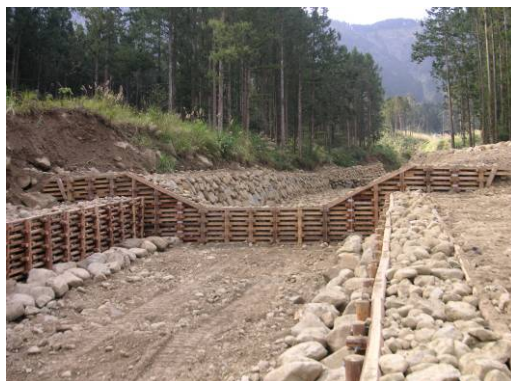
a) sabo dam made of Japanese Fir just finished on Feb 8 2006 b) after the heavy rainfall event on Jun 26 2006
