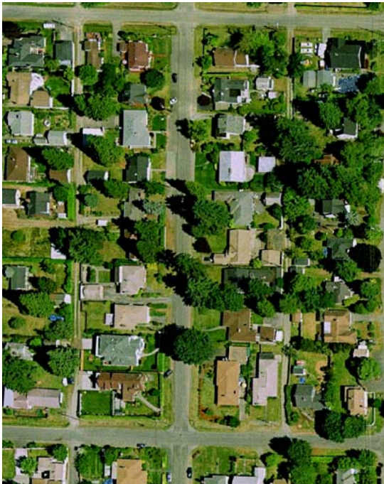
Figure 1. Seattle Streets – Before Construction
