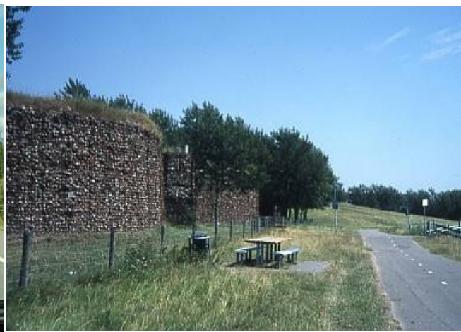
Figure 5. Innovative noise barrier at a resting site on a Dutch motorway, providing both noise protection and habitat. (H.v.B.)
