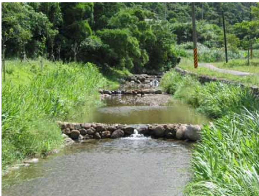
Fig. 5 Typical Grade control Structure
