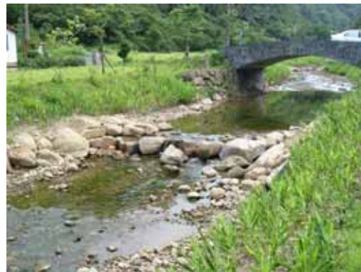
♦ Restored No.8 Grade control structure
