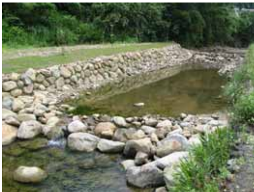
♦ Restored No.2 Grade control structure
