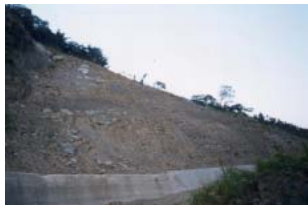
Figure 8. Highway No. 149 A, 28K+120, Before Construction
