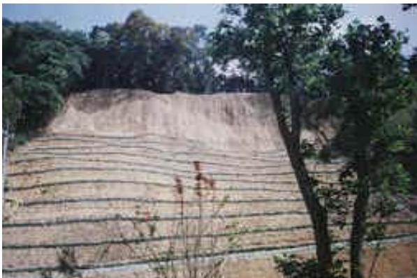
Figure 4. Provincial Highway No. 3, 80K+100, Spreading Grass Seeds to Cover the Slope
