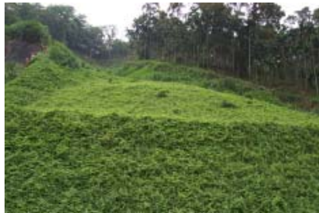
Figure 13. Status of Highway No. 110, 32K+700 after Construction
