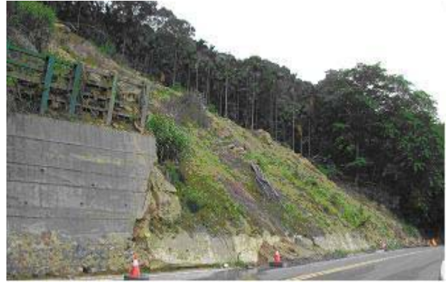
Figure 12. Status of Highway No. 110, 32K+700 under Construction
