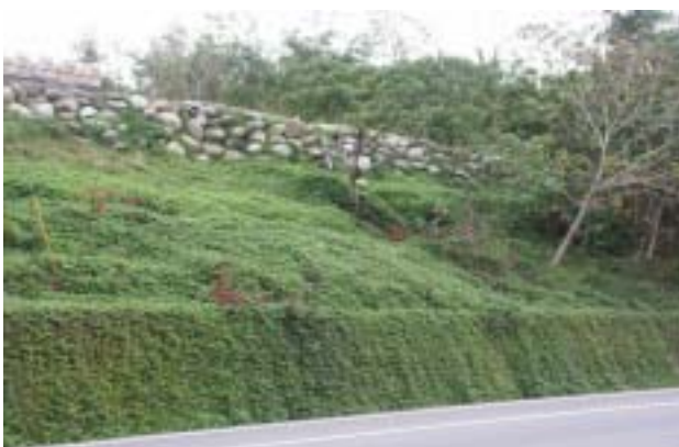
Figure 11. Provincial Highway No. 11, 154K, Stabilizing the Side Span with Plant-cultivation
