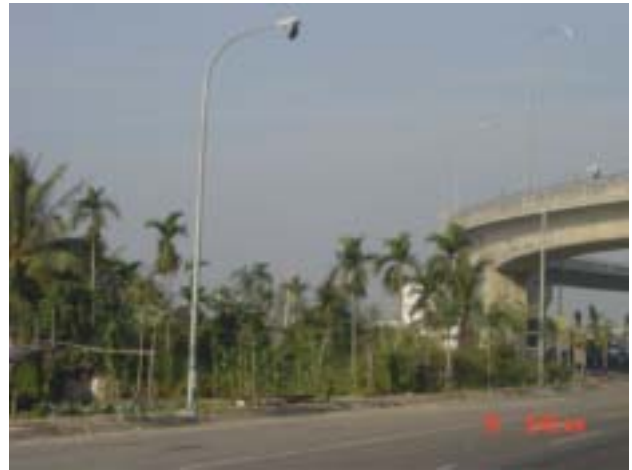
Figure 26-27. Provincial Highway No. 88 Wan-Dan Interchange, Street lights equipped with lampshades to avoid affecting growth of crops
