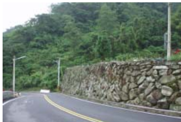
Figure 14. Highway No. 149, 54K, Side Slopes with Dry-stone Masonry
