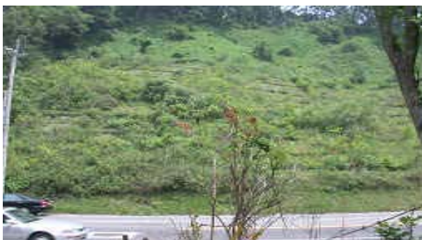
Figure 5. Provincial Highway No. 3, 80K+100, One Year after Construction
