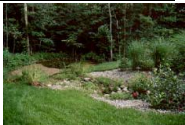
Figure 2. Typical 'Rain Garden' Bioretention System
