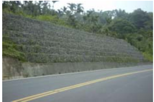
Figure 18. Provincial Highway No. 18, 28K, Construction for Gabion Slope Protection
