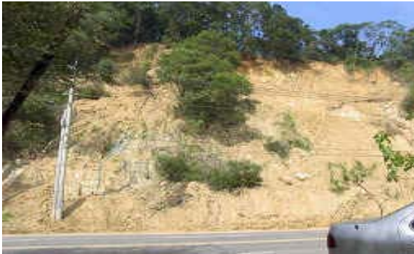
Figure 3. Status of Provincial Highway No. 3, 80K+100, Before Construction
