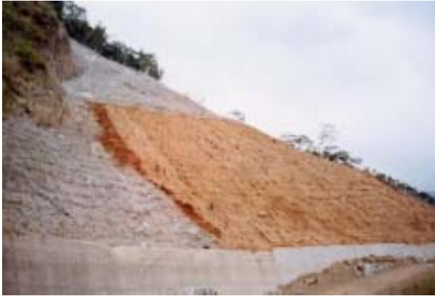
Figure 9. Highway No. 149A, 28K+120, Piling, Fencing, and Plant-cultivation
