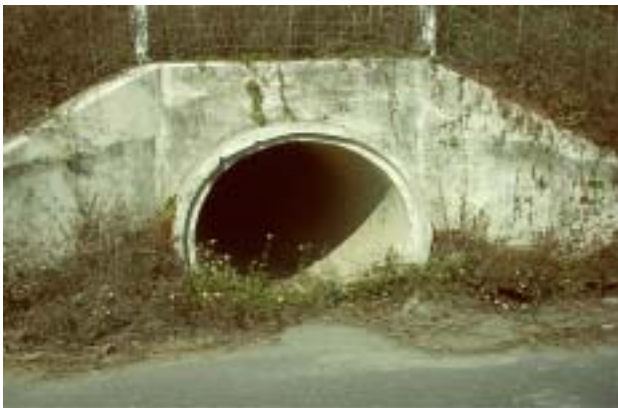
Figure 21. Provincial Highway No. 78, Taixi-Kuken Section, Box (Tube) Culvert with Courses for Living Beings
