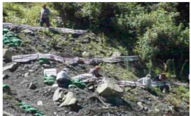
Figure 7. Piling and Fencing at Provincial Highway No. 21, 119K
