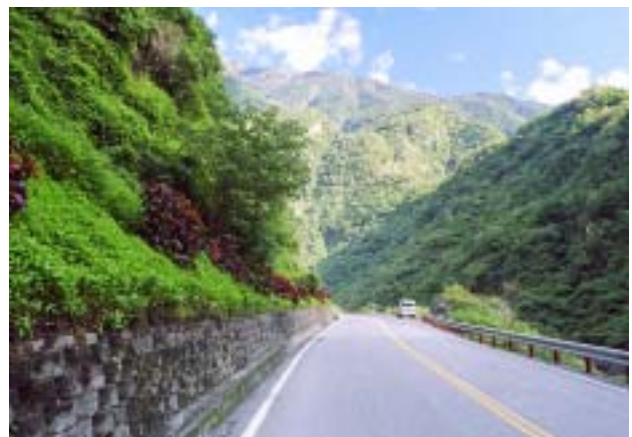
Figure 23. Provincial Highway No. 8, 182K+200, Side Slopes Piles with Bricks; Structural Height is Lowered; Vines and Colorful Bushes beautify the road
