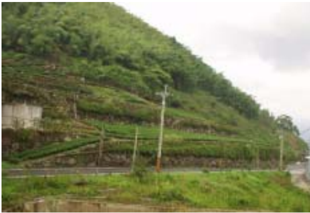
Figures 15-16. Route 169, 10K-12K A Ladder-style Slope with Dry-Stone Masonry
