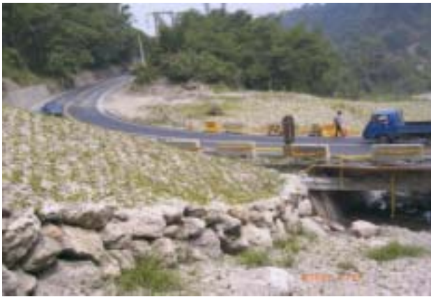
Figure 17. Route No. 172, Dry-stone Masonry at the Headstream of Chong Chong Bridge
