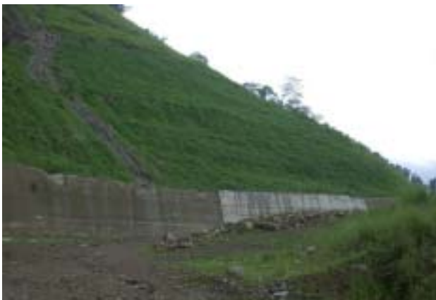
Figure 10. Status of Highway No. 149 A, 28K+120, After Construction
