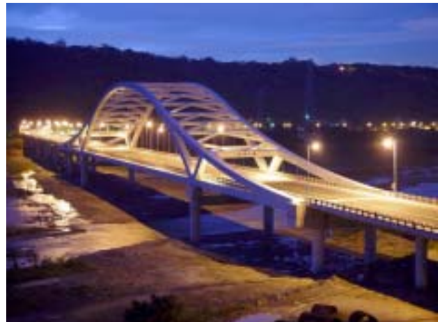
Figure 19. Provincial Highway No. 4, Kanjin Bridge
