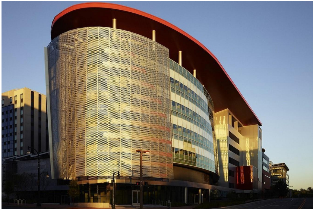
The building envelope of The Unisphere
