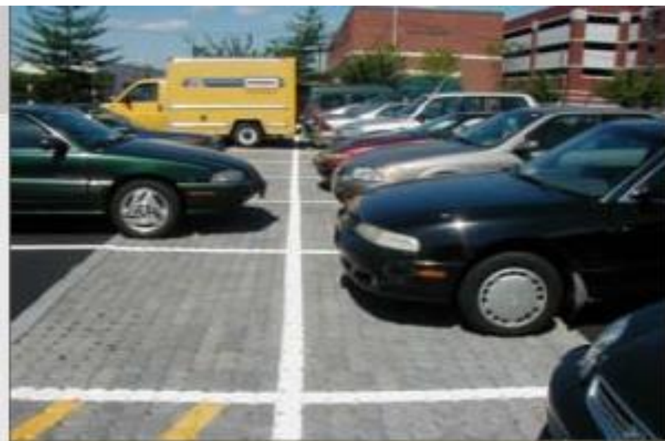
Porous pavement covers about 1/3 of each parking space in the D.C. Navy Yard parking
