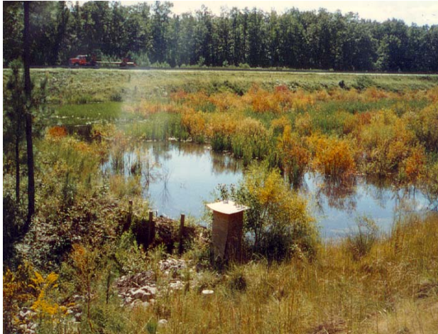
Figure 5. Constructed Wetland in a Highway Medium
