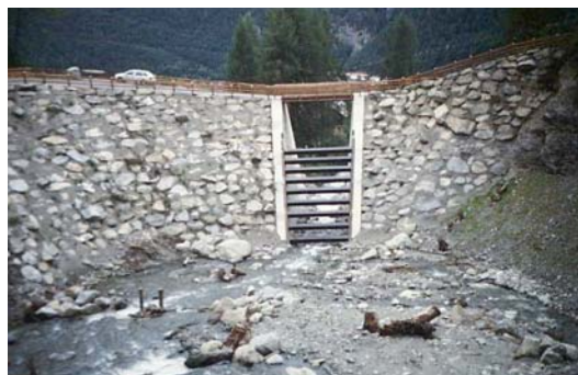
Fig. 16. Debris retention basin with special outlet construction (beam dam) just finished.
