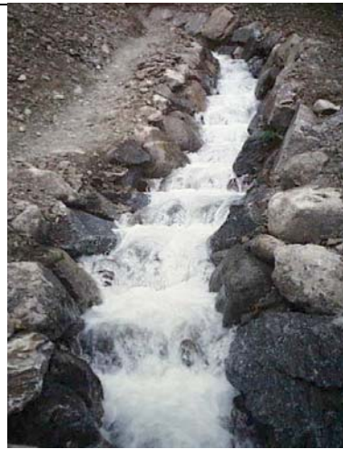
Fig. 17. The above debris retention basin is by-passed by a channel with water for running a sawmill. The channel was reconstructed using dry-laid stones and timber logs as foundation.
