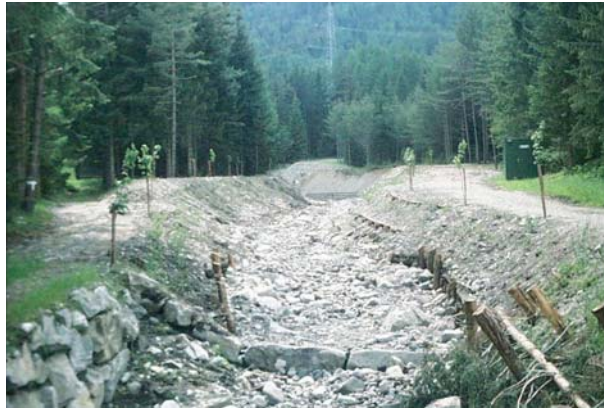
Fig. 10. Torrent reach with concrete sills (covered by sediment) and dry-laid stone crowns, fixed by steel cables (upstream the sills, therefore not to be seen), the bank protection is done by different soil-bioengineering methods, just after implementation
