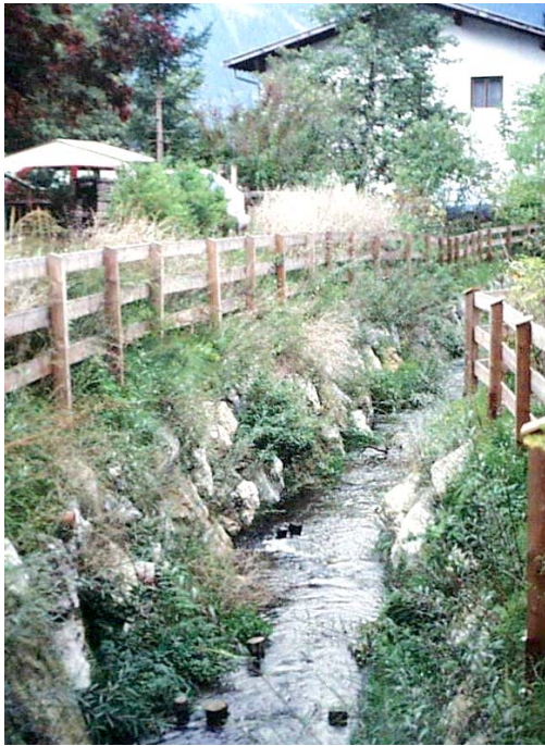
Fig. 12. Channelwork controlling a small stream in a settled area. The stream bottom is fixed by low sills as shown in Fig. 2., the banks are protected by walls made of dry-laid stones.
