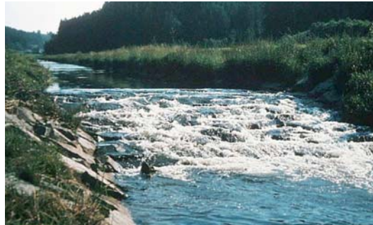
Fig. 15. Ramp of dry-laid stones as alternative to a dam or sill in a large flood stream.
