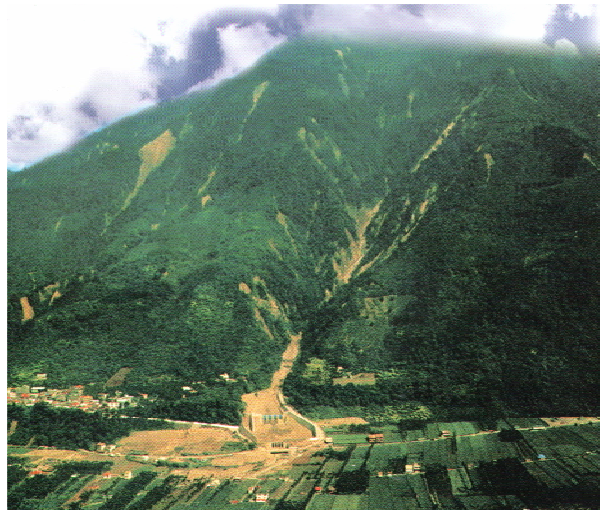
Fig. 5. Example from Taiwan. Project Feng Chu. In the upper reach till down to the debris flow retarding basin, debris flows may occur. Natural orientated works only can be done on the slopes with soil bioengineering works but not in the torrent itself. Below the street, where the energy level is lowered, between the houses and at the agricultural area nature orientated works can be done – when you can acquire the space.
