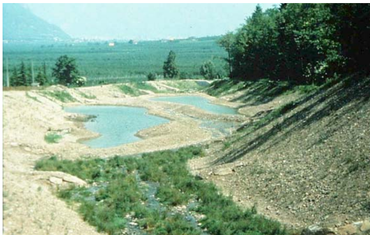
Fig. 18. and Fig. 19. Debris retention basin shortly after excavation and 5 years later. ( Southern Tyrol, Italy)
