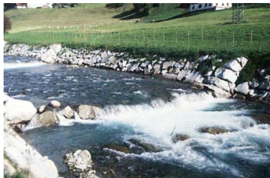
Fig. 14. Control works in a large bed-load transporting stream by sills made of dry-laid stones concrete foundation and fixed by steel anchors and by low revetments made of dry-laid stones.
