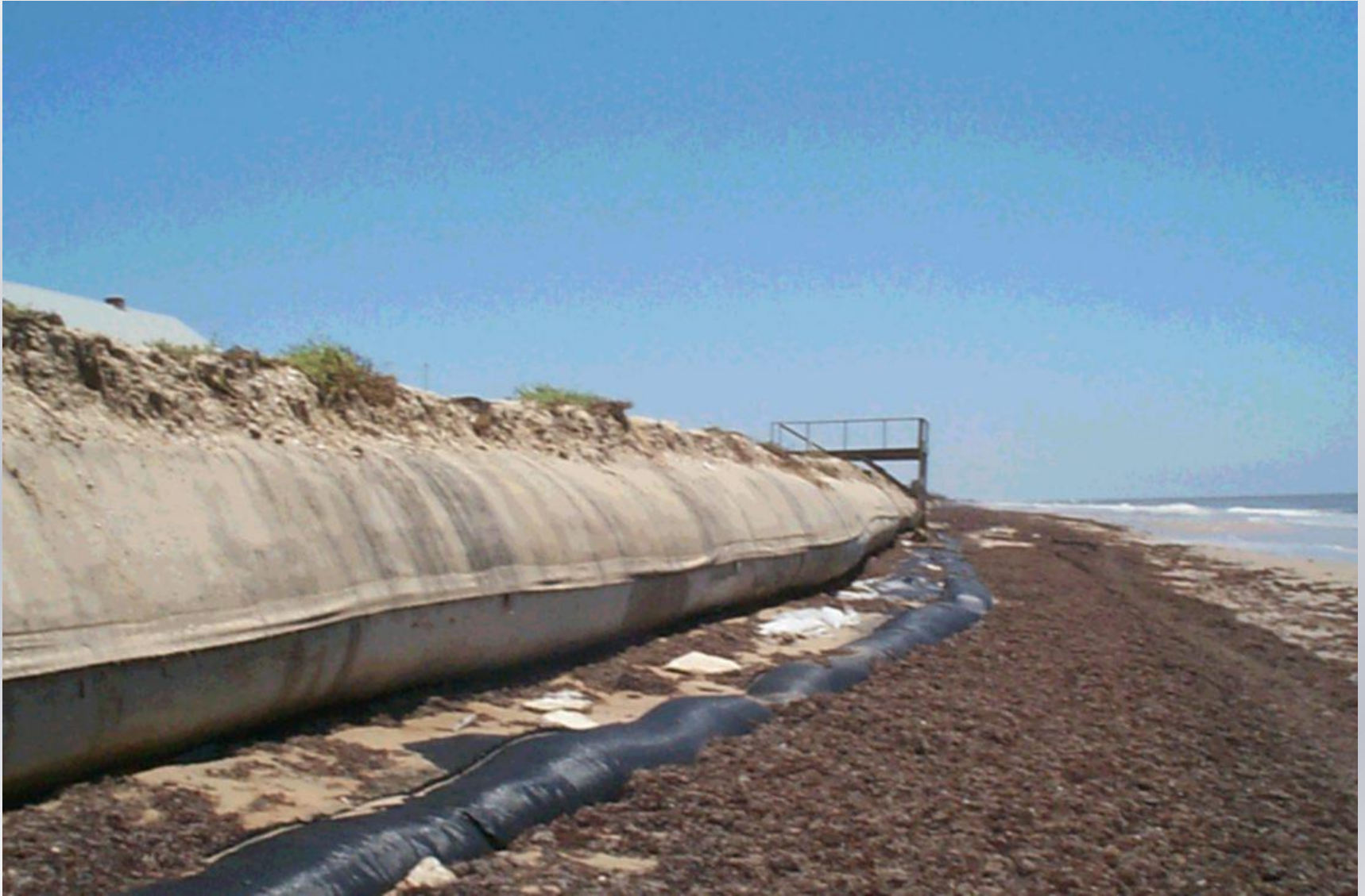
Geotextile Tube as dike/dune core; Source: C-Horse Construction
