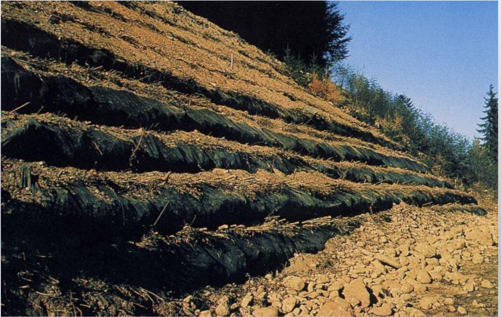
Geosynthetic reinforced river embankment, Worb, Switzerland; Source: Schiechl, Stern
