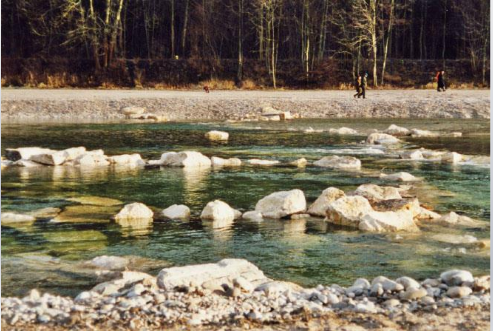
River Isar, near Munich, bed ramp after renaturation; Source: BLK
