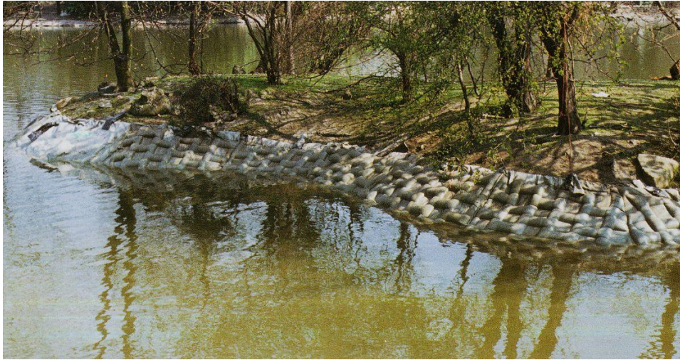
Geosynthetic Mortar and Sand Mattresses; Source: Huesker Synthetic
