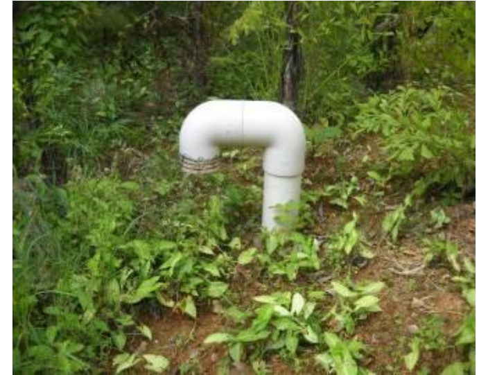
地下雨水蓄水池 Underground stormwater storage tank
