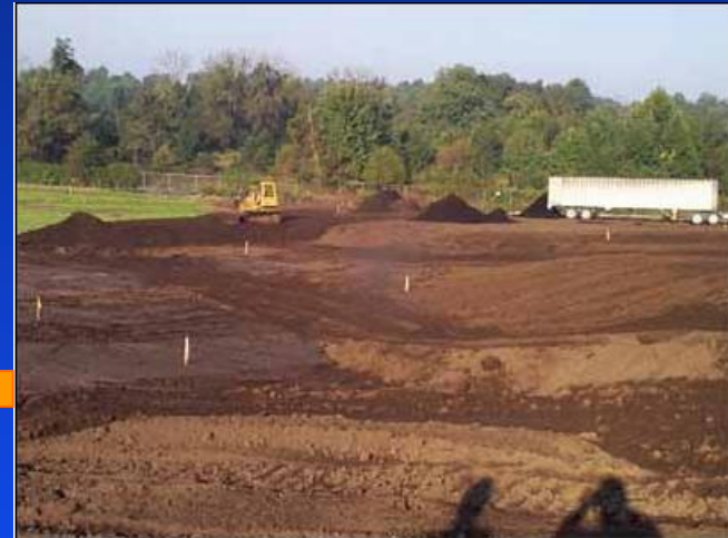
Southern Maryland Wood Treating Site: On-Site Thermal Desorption of Contaminated Soils, Final Grading and LeafGro Placement
