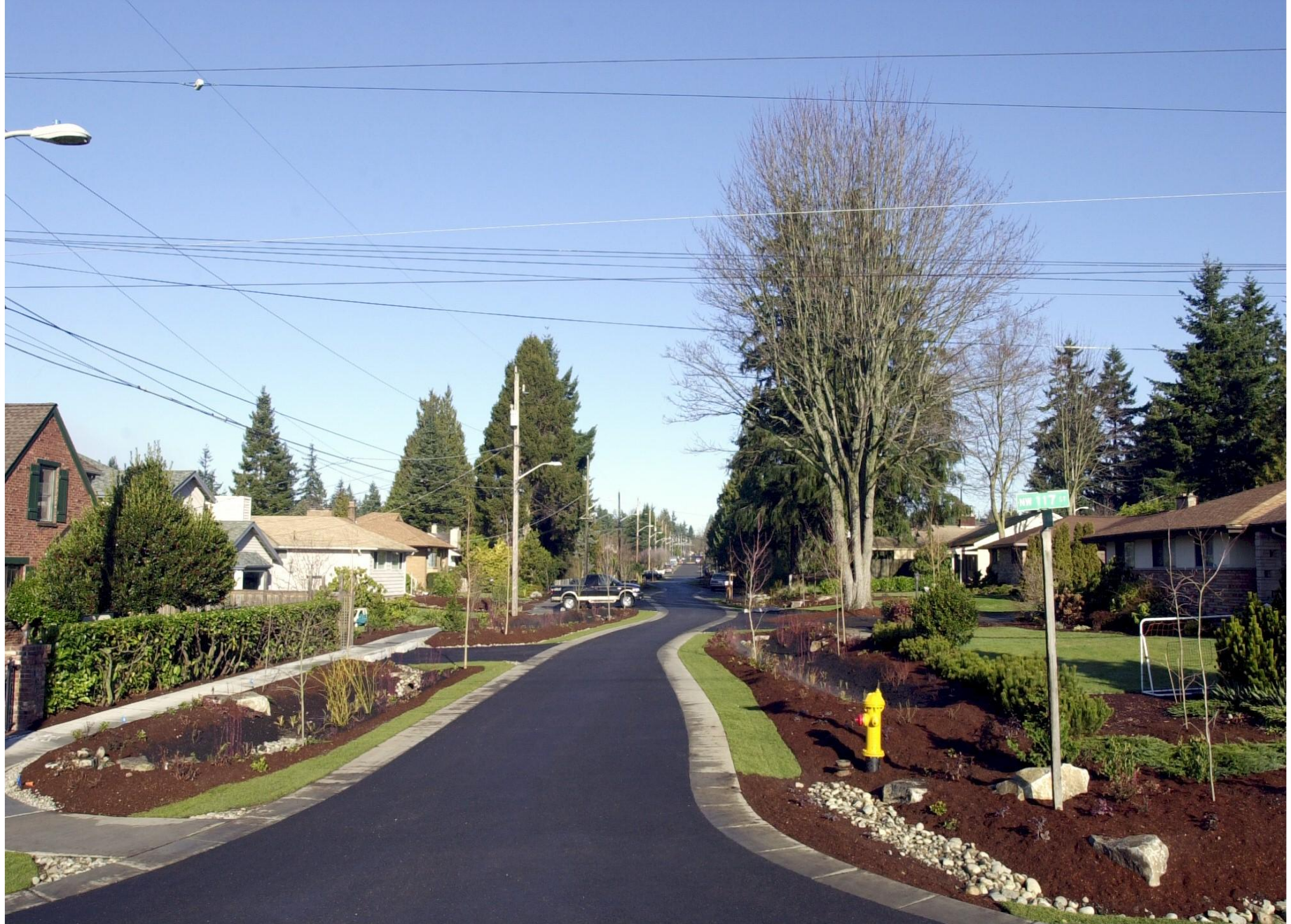
After Completion - January 2001
