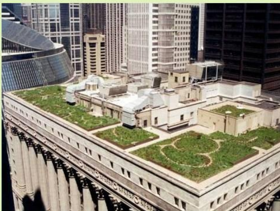
City Hall Rooftop Garden (Intensive System)
