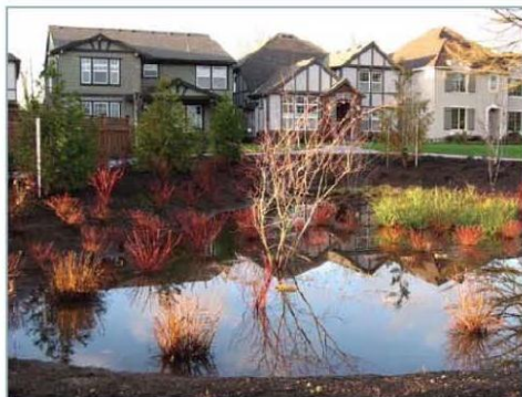
Figure 2: Decentralized stormwater management features, such as this bioretention area in the Villobos project, collect runoff from rooftops, sidewalks, and yards for infiltration into the ground below.
