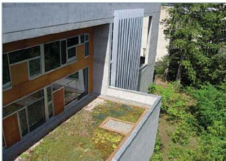
Figure 1: A green roof at Evergreen College was built to offset the addition of new impervious surfaces from new parking spaces.
