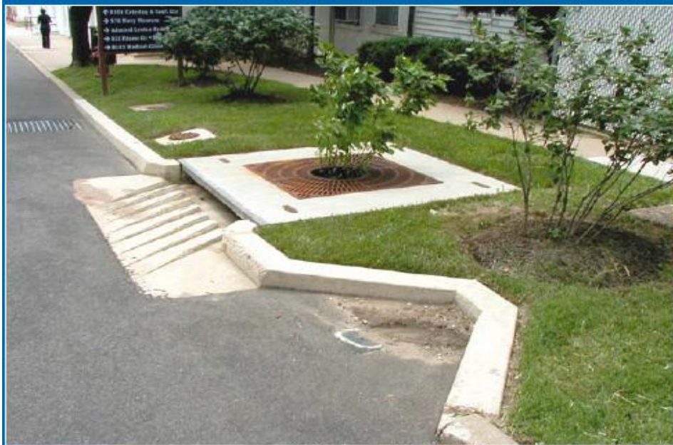
Tree box filter at the Washington, DC Navy Yard
