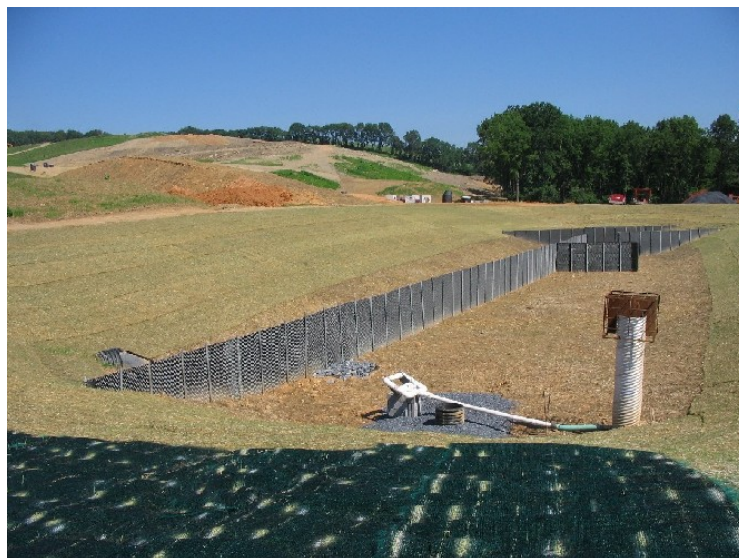
溢流管式排水沉砂池 ( http://www.northamptoncd.org/ )
