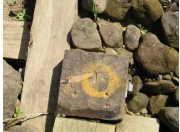
Figure 9. Monitored points with marked nails on the joints of wooden structure at No.1 site
