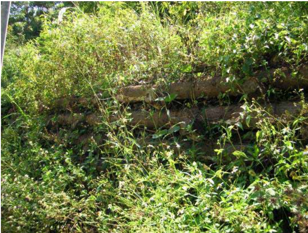
Figure 3. Retaining wall at No.2 site, Shan-An, Shueili.
