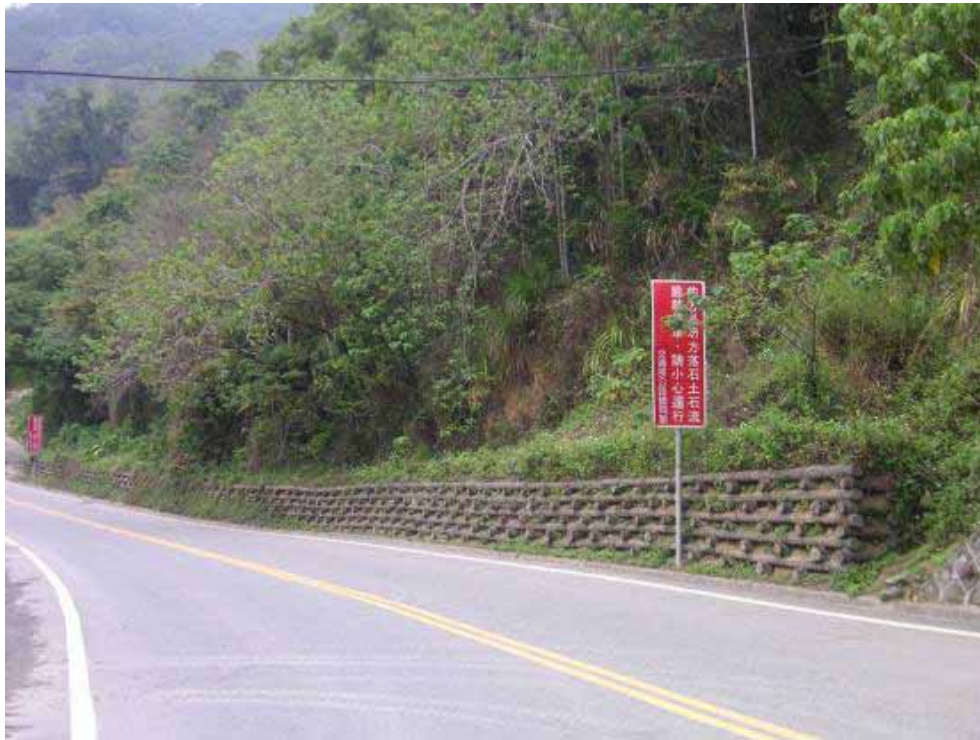
Figure 6. Retaining wall at No.5 site, Ming-He, Shueili.
