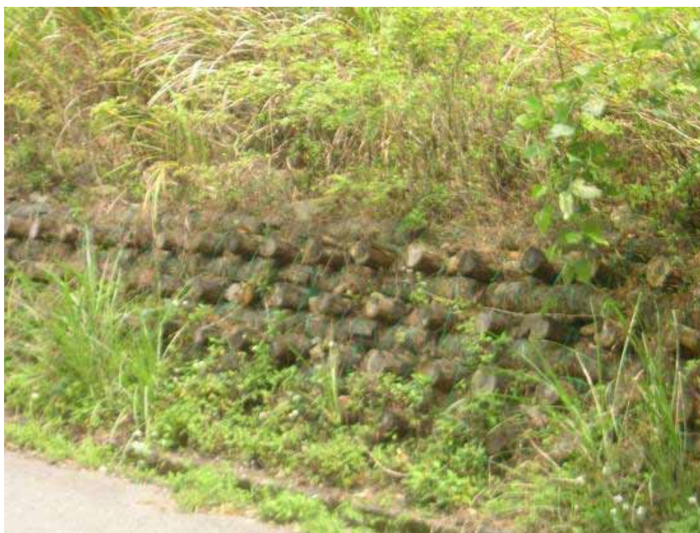
Figure 5. Retaining wall at No.4 site, Ren-Lun, Sinyi.
