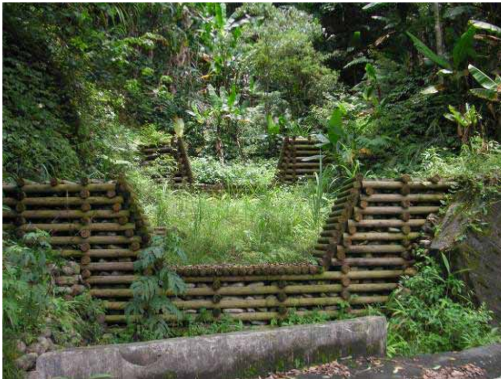
Figure 7. Check dam at No.6 site, Datong, Yilan.
