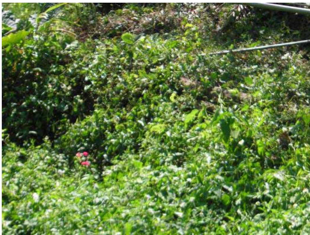
Figure 4. Revetment along the creek at No.3 site, Shan-An, Shueili.
